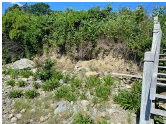
Photo 1 & 2 – Images depicting how the toe of slope has been undercut and compromised.
