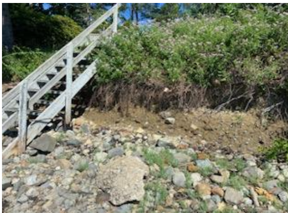
Photo 1 & 2 – Images depicting how the toe of slope has been undercut and compromised.
